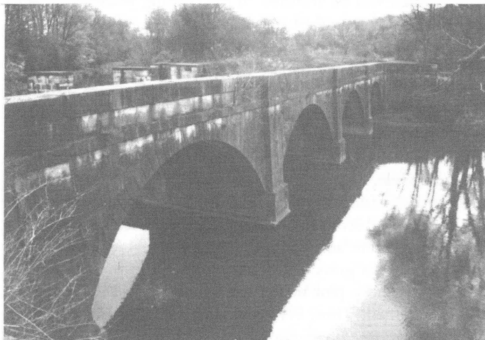
Erie Canal Aqueduct at Camillus New York. The trunk was formed by a wooden trough that rested on the piers in photo on right.
