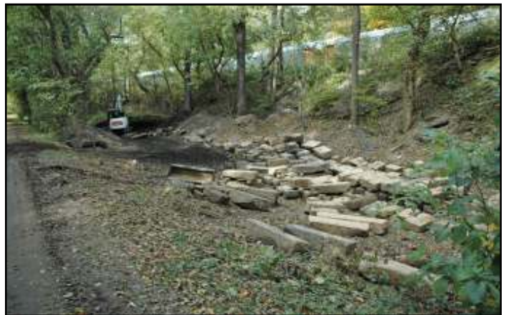
Above: Hundreds of the original cut stones used to build the Catoctin Aqueduct in 1832-34 were recovered from Catoctin Creek and buried after the Aqueduct collapsed in 1973. Recently the stones were recovered from the canal prism east of the Catoctin Aqueduct site. Shown here are less than half of the stones recovered thus far.
