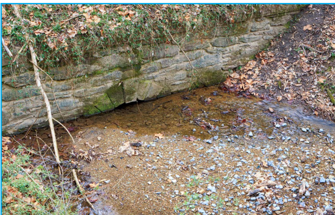
Filled culverts, as shown at left, pass a limited amount of water and can allow water build-up during high water conditions that can present a risk to the towpath and prism. Open culverts, as shown on right, protect the integrity of the canal as they have done for 165 or more years. With the help of the VIPs there soon will be more open culverts. Photos by Steve Dean.
