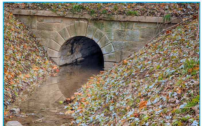
Filled culverts, as shown at left, pass a limited amount of water and can allow water build-up during high water conditions that can present a risk to the towpath and prism. Open culverts, as shown on right, protect the integrity of the canal as they have done for 165 or more years. With the help of the VIPs there soon will be more open culverts. Photos by Steve Dean.
