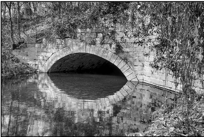
Culvert 136, with its 20-foot span, is a fine example of culvert construction and is worth a quick stop. It is just over a half mile below Dam 5.
