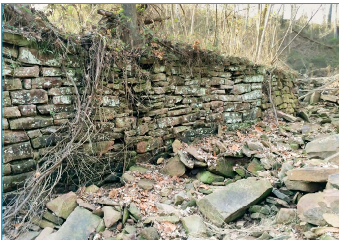
A close-up of the northern section of the Bull Run retaining wall. Even this intact section shows signs of distress: stones have fallen out of the wall, and trees and vines are growing into it, further weakening the structure. Photo by Garrett Peck.
