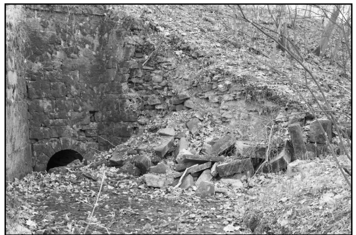
The recently collapsed berm wing wall at Culvert 141.
