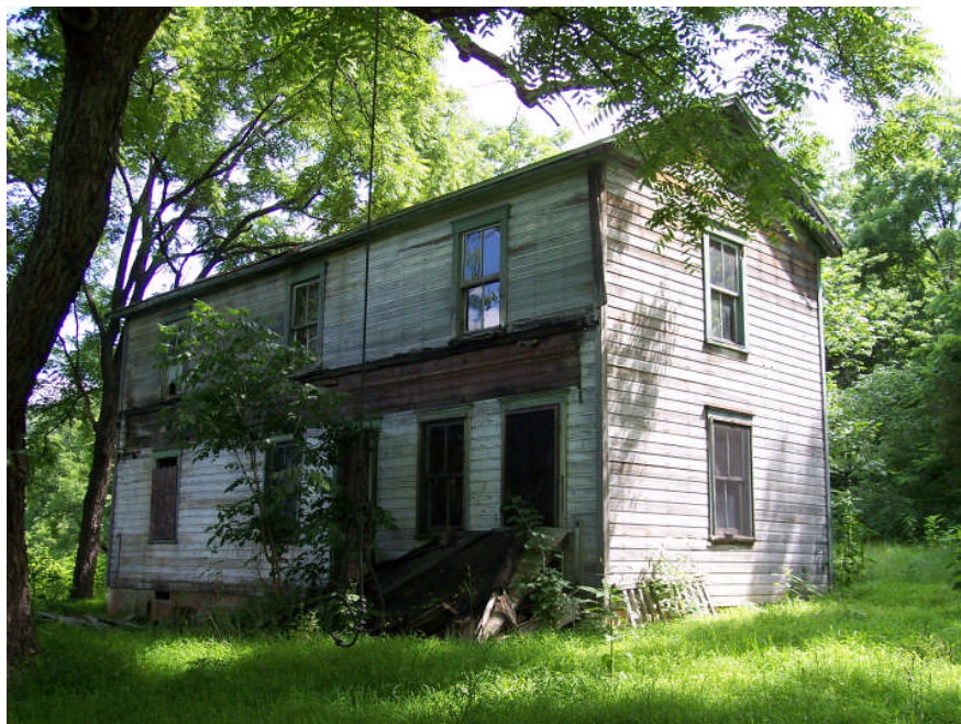
By 2009, the front porch floor and roof had fallen down as shown above. Rotating our view to the right, the Raymond Higgins house comes into view as shown:
