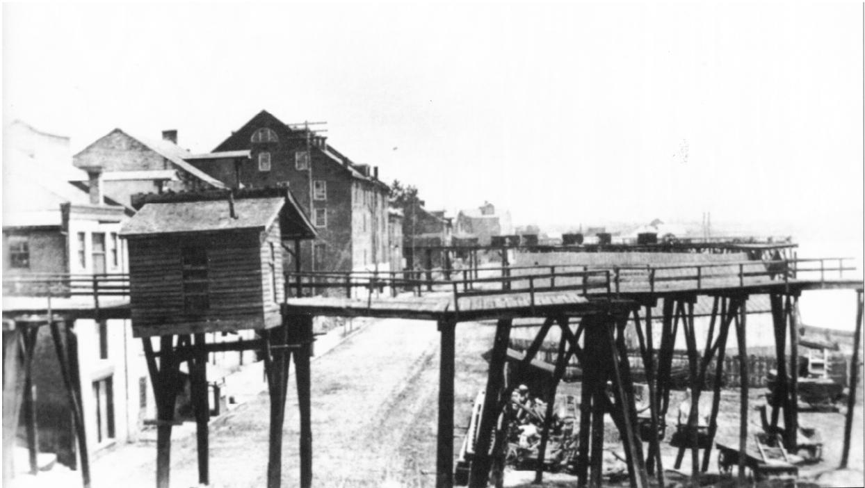
The above photograph, also from the National Park Service, shows one of the trestle works which were used to transfer coal by hand car from the canal, to the left, to the coal yard or sailing vessel at a wharf, on the right.
