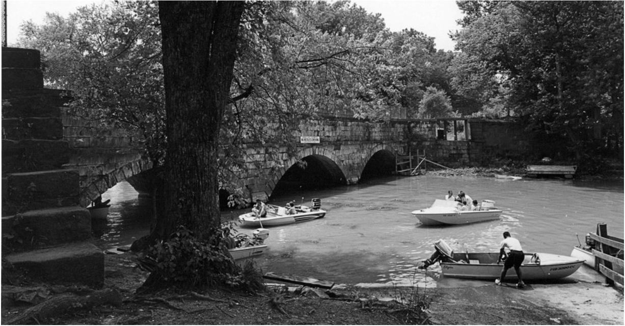
Approximately Sept. 11, 1971 a localized storm sent flood waters surging down Seneca Creek. The high water and debris resulted in the failure of the western arch of the aqueduct. In the photograph below, Park Service personnel standing on a float under the middle arch were
