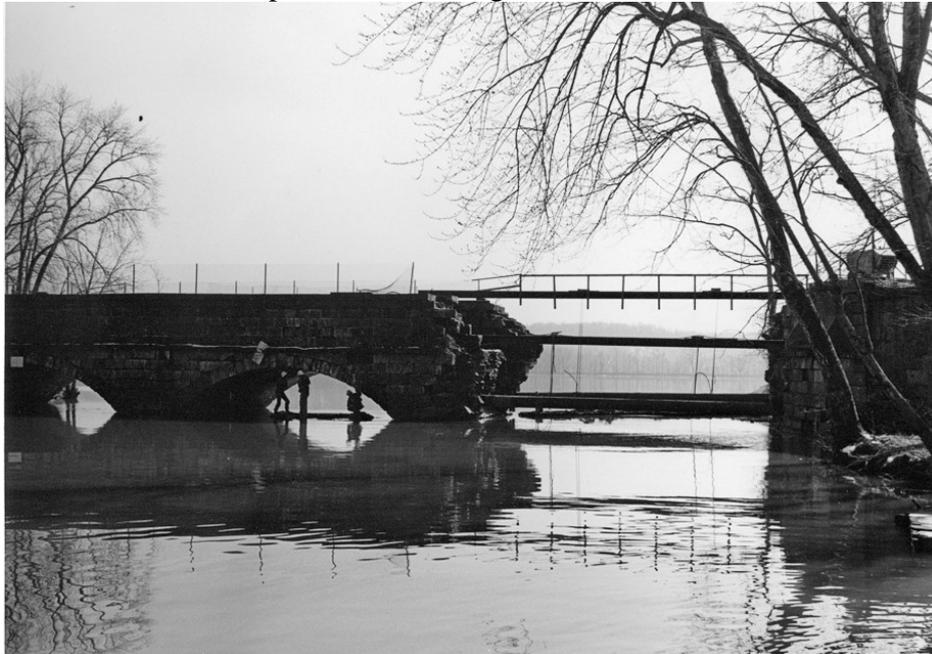
examining it for damage. The circular steel braces were already in place, as was the footbridge spanning the missing arch. Subsequently "Shotcrete" was applied to the exposed surfaces to protect them from the weather and further deterioration. The following photograph was taken
