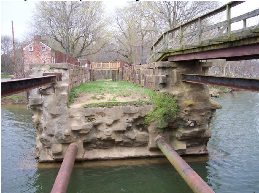
The above photograph was taken by the author in 2009 and illustrates that the application of "Shotcrete" has minimized further deterioration of the face of the fallen arch. Without the braces, the weight of the structure might have caused it to shift toward the viewer and thus jeopardize the integrity of the middle arch. The wooden pedestrian footbridge across the lock
